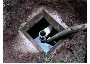
**WARNING:** If the liquid level in the tank is above the top of the filter, pump the tank prior to removing the filter cartridge.
